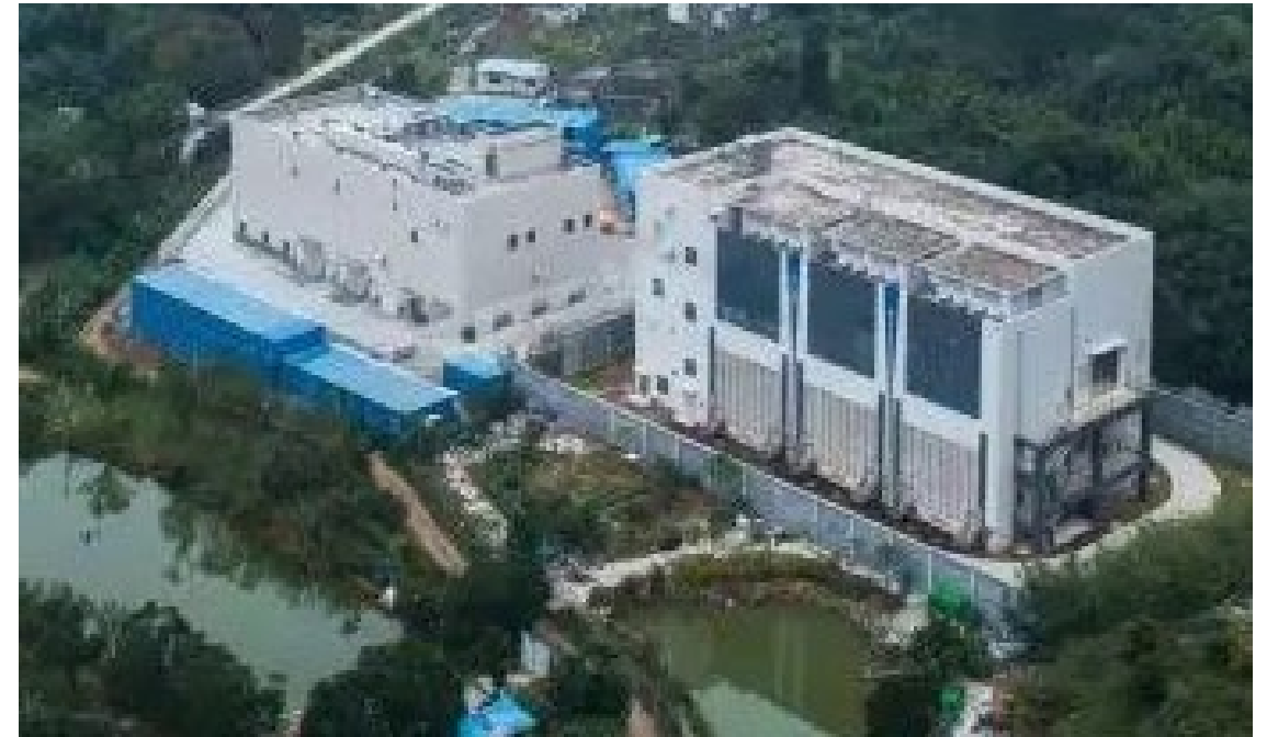
Demonstration project in Tangjiawan, Zhuhai, (珠海唐家湾示范工程)
